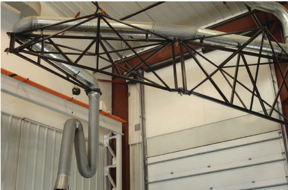
Custom PAC, 32' Double Articulation, High Temperature Hose Drop
